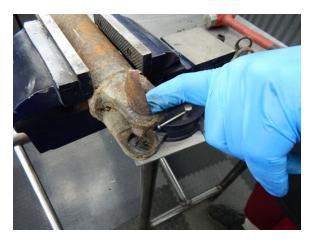
Clean away any rust, nicks, or debris from the drive shaft yoke and the flange yoke, using fine emery cloth or sand paper.
