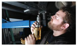
**7.** Install the self-drilling flat head screws with a drill and a Phillips #2 bit until it's flush with the surface.
